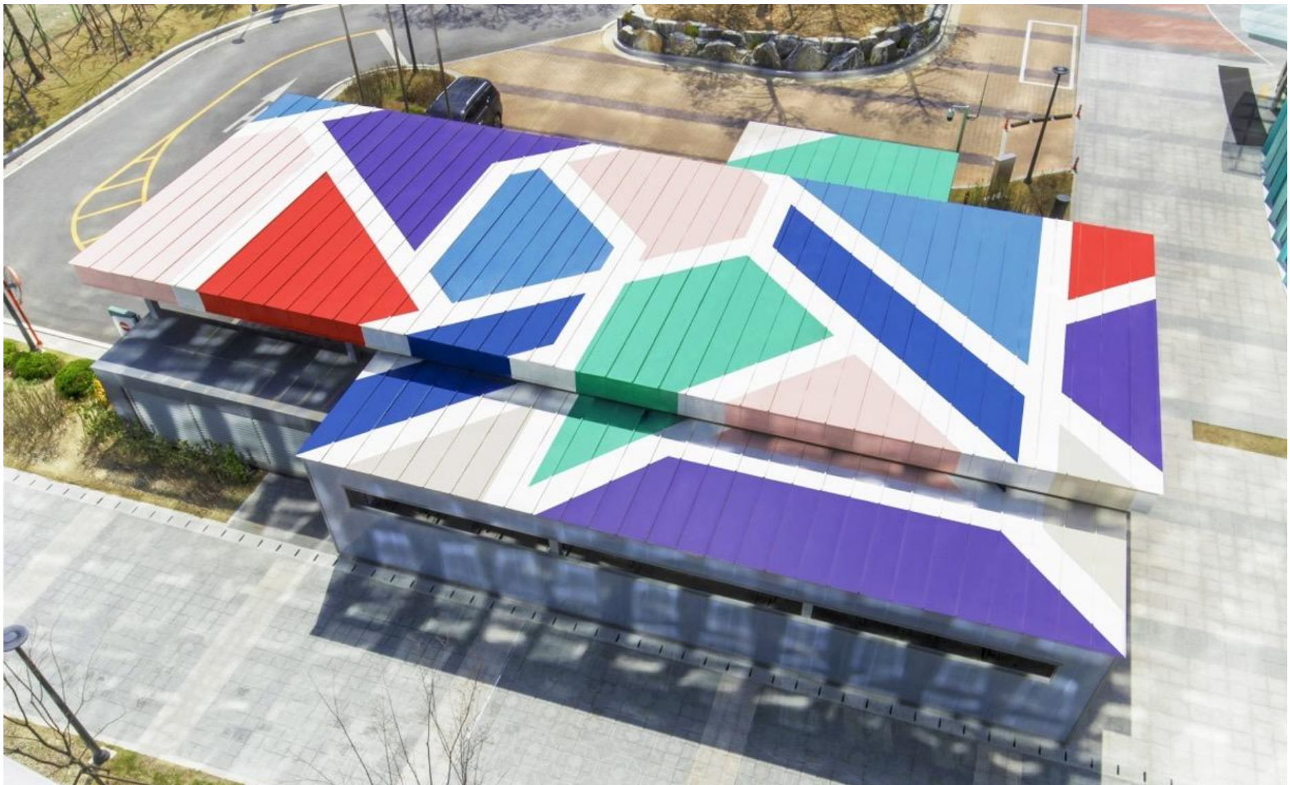
Rooftop Painting Hana Bank, South Korea 2017
